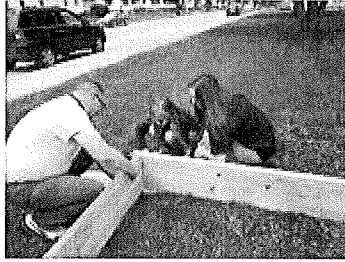
PUTTING TOGETHER THE FRAME
